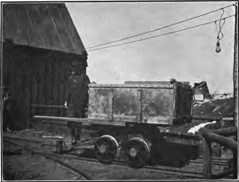
FIGURE 4 TOP-TRAM CAR, SALISBURY MINE
